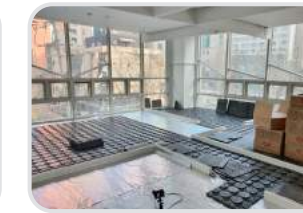
Shop and Office
